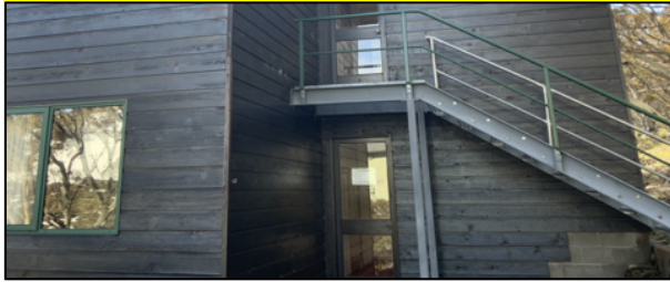
Figure I - Balustrade to Stair Incorporates Openings which allow for a 150mm Sphere to Pass Through.
