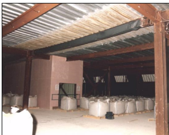
Figure 30 - Cardington Fire Test - British Test 1 - Buckling of Beam at Protected/Unprotected Interface.
